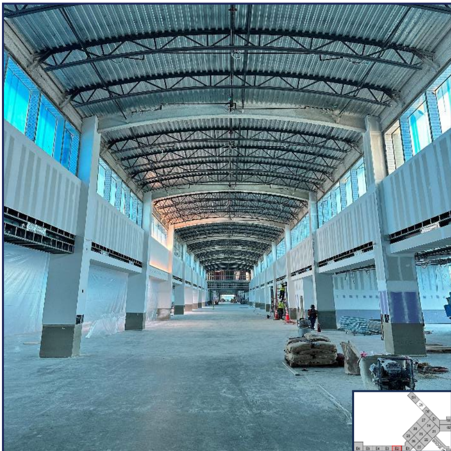
Drywall Finishing in Zone E2 of Concourse E
