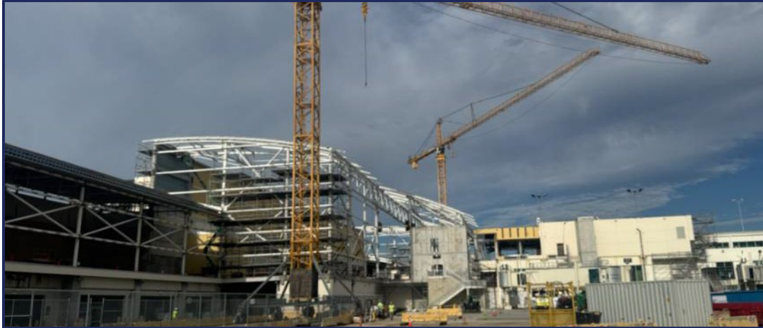
Central High Barrel Roof - Truss and Eyebrow Installation
