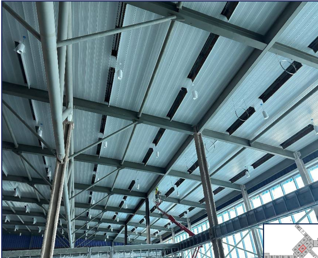
Installation of light fixtures in Zone 25 of the Main Terminal
