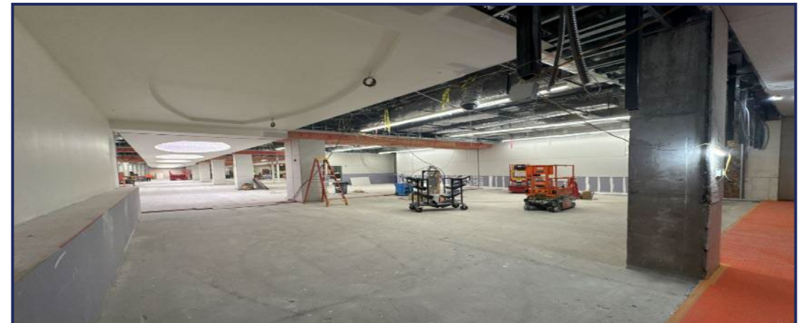
East Side Consolidated Check – Framing and Drywall
