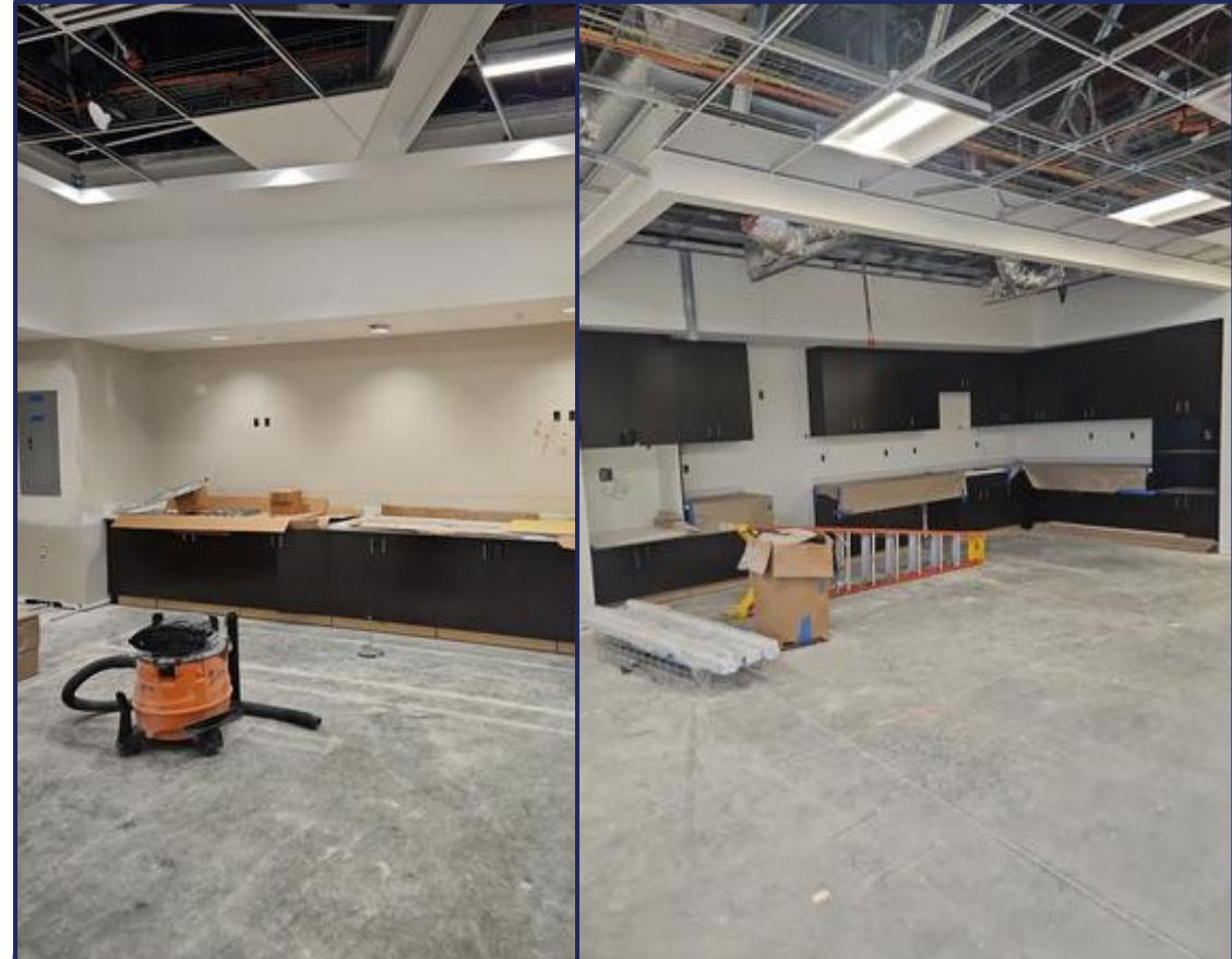
Millwork was installed throughout the building.
