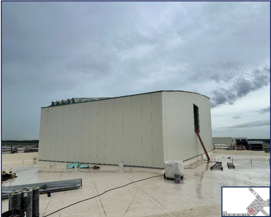
Installation of insulated metal panels for the Mechanical Penthouse in Zone 26 of the Main Terminal.
