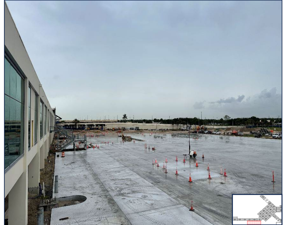
Installation of Concrete Apron South of Concourse E
