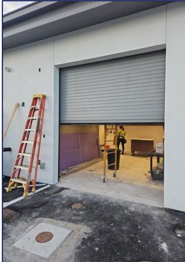
The overhead door to the sallyport was installed.
