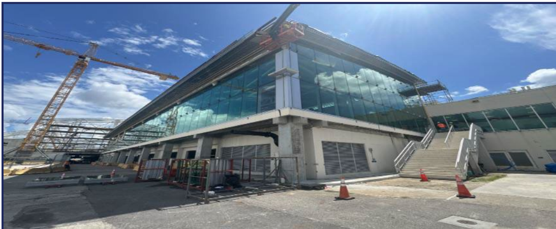
Curtainwall Erection Ongoing on West side of Terminal Building
