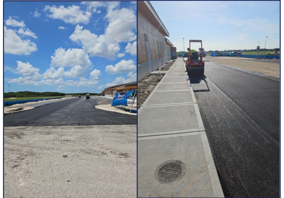
The first lift of asphalt paving was completed.
