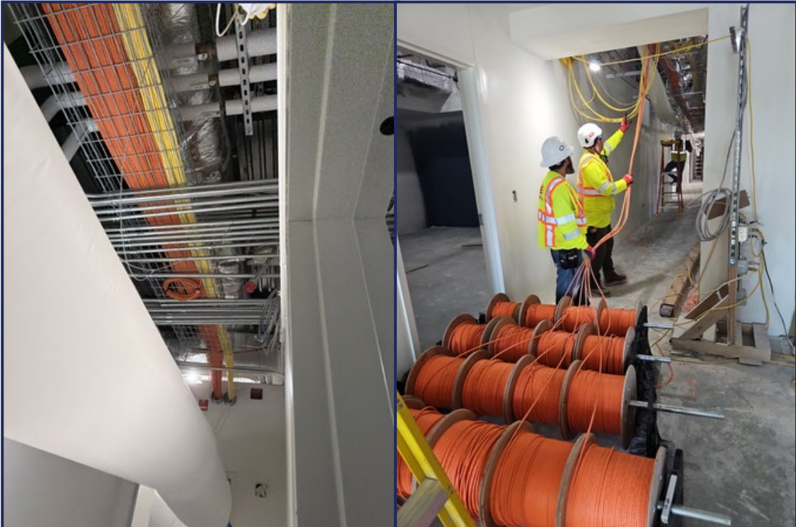
Cable trays were installed and low voltage cabling was pulled throughout the building.
