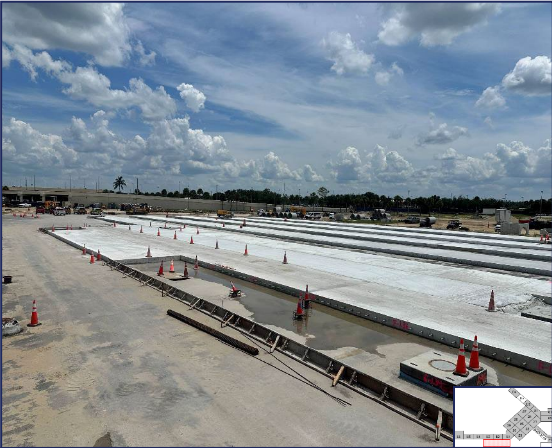
Installation of Concrete Apron south of Concourse E.
