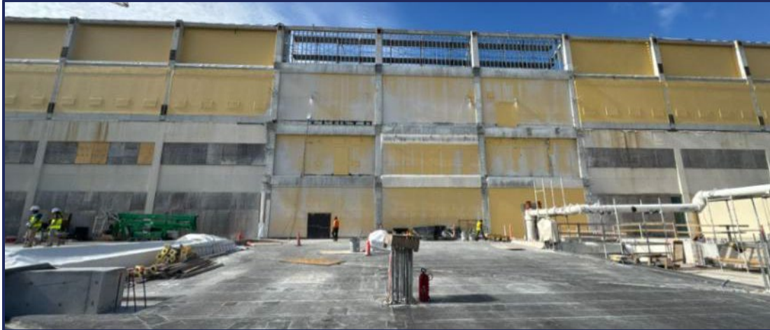
Concourse C Partial Demolition in Progress
