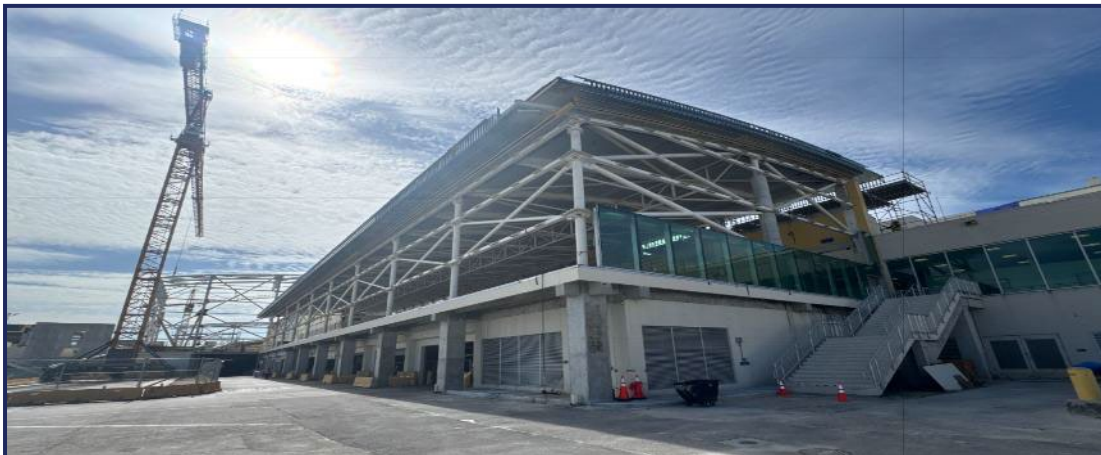
Curtainwall Erection started on West side of Terminal Building
