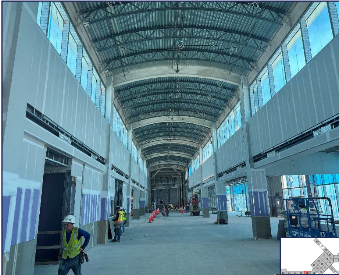
Drywall Installation in Zone E2 of Concourse E.
