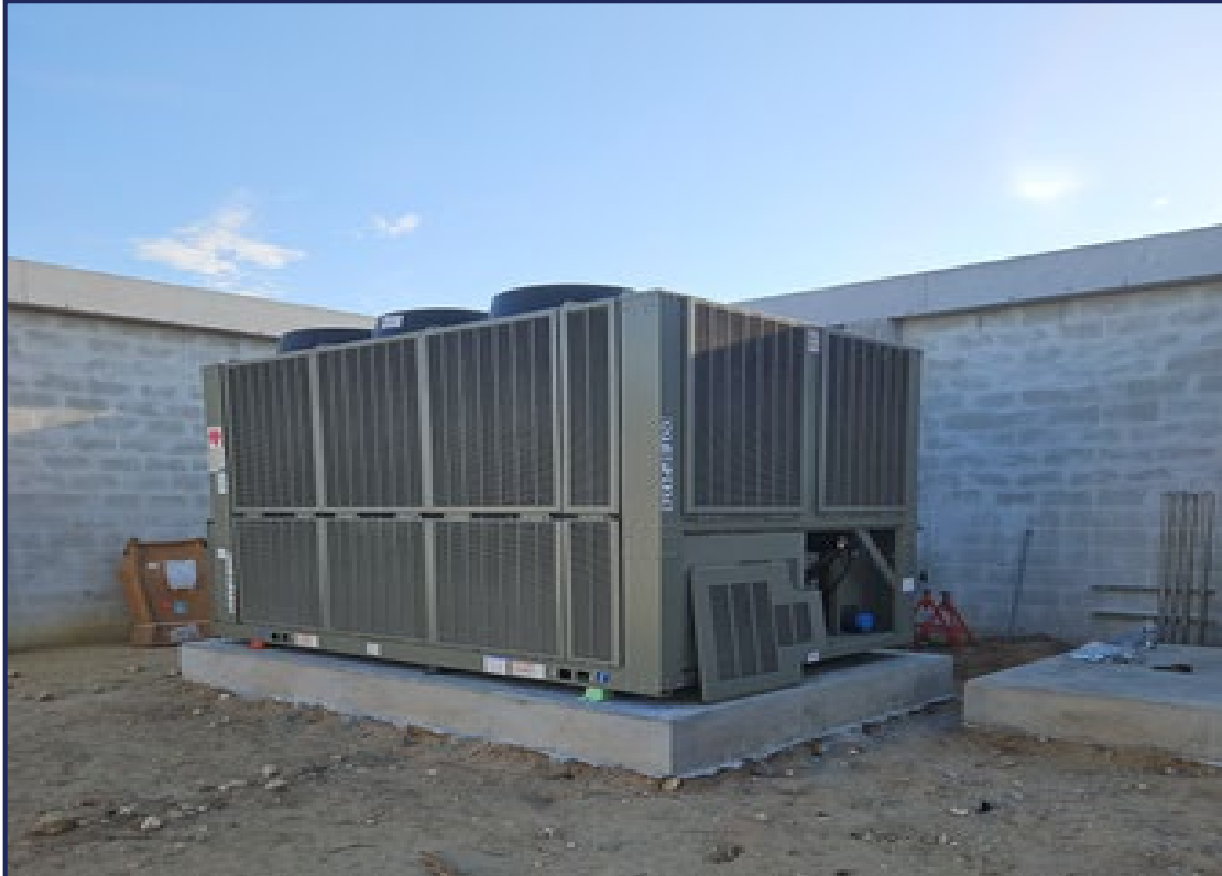
The mechanical chiller was set in the mechanical yard.
