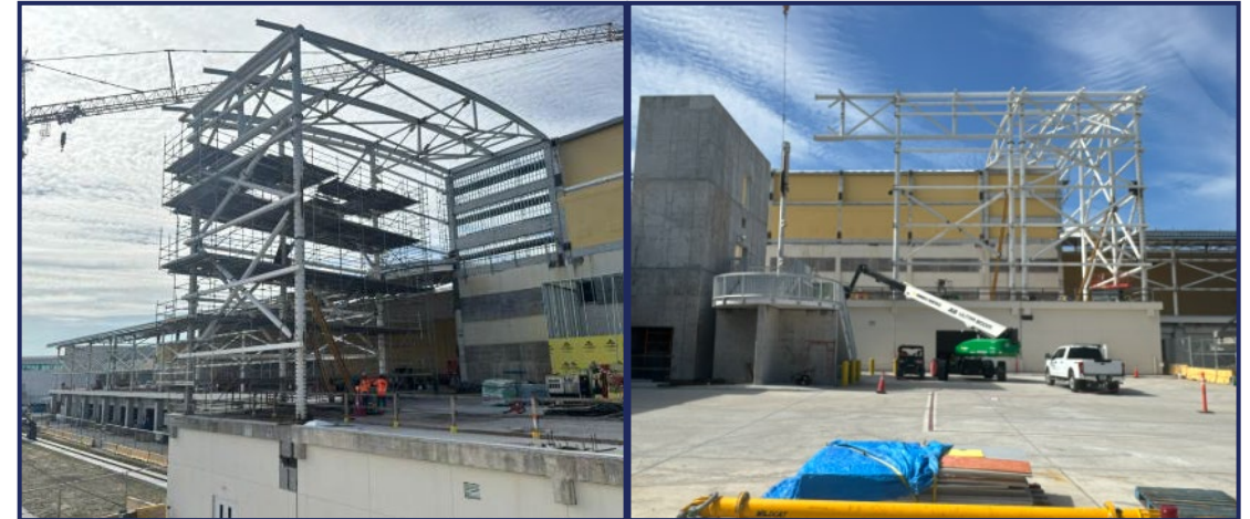
East and West High Arch Roof Trusses - Erection progressing
