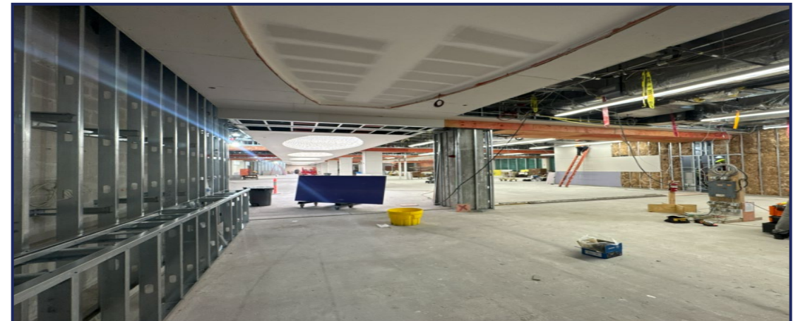
East Side Consolidated Checkpoint – Framing and Drywall
