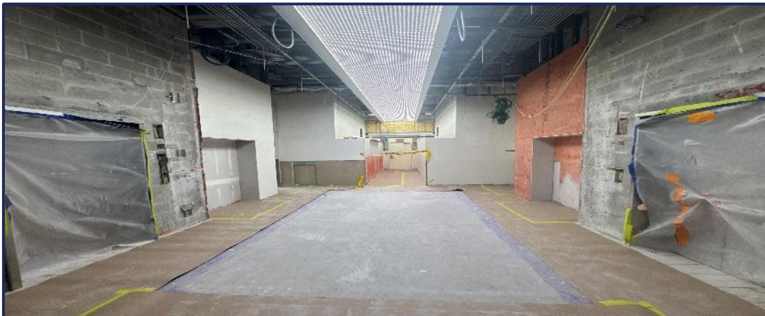
Elevator 8 & 9 Lobby (2nd Floor) to LCPA Admin Offices in Progress
