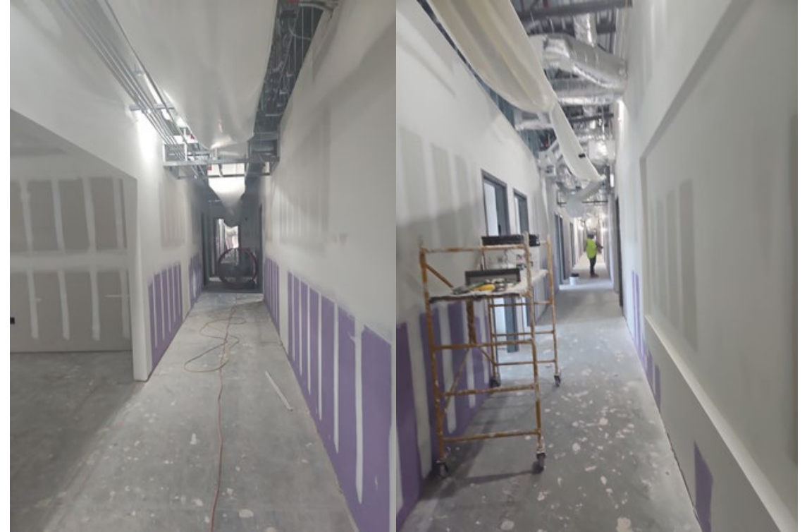
Hanging of drywall was completed for interior walls.
