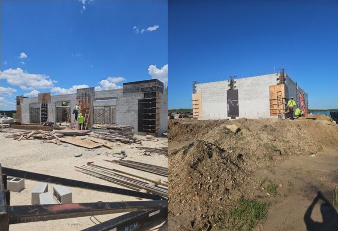
Masonry blockwork at the mechanical yard in progress.
