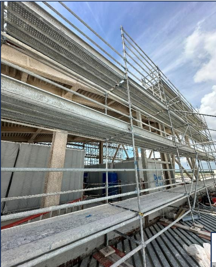
Fire Spray for the mechanical penthouse in Zone 26 of the Main Terminal
