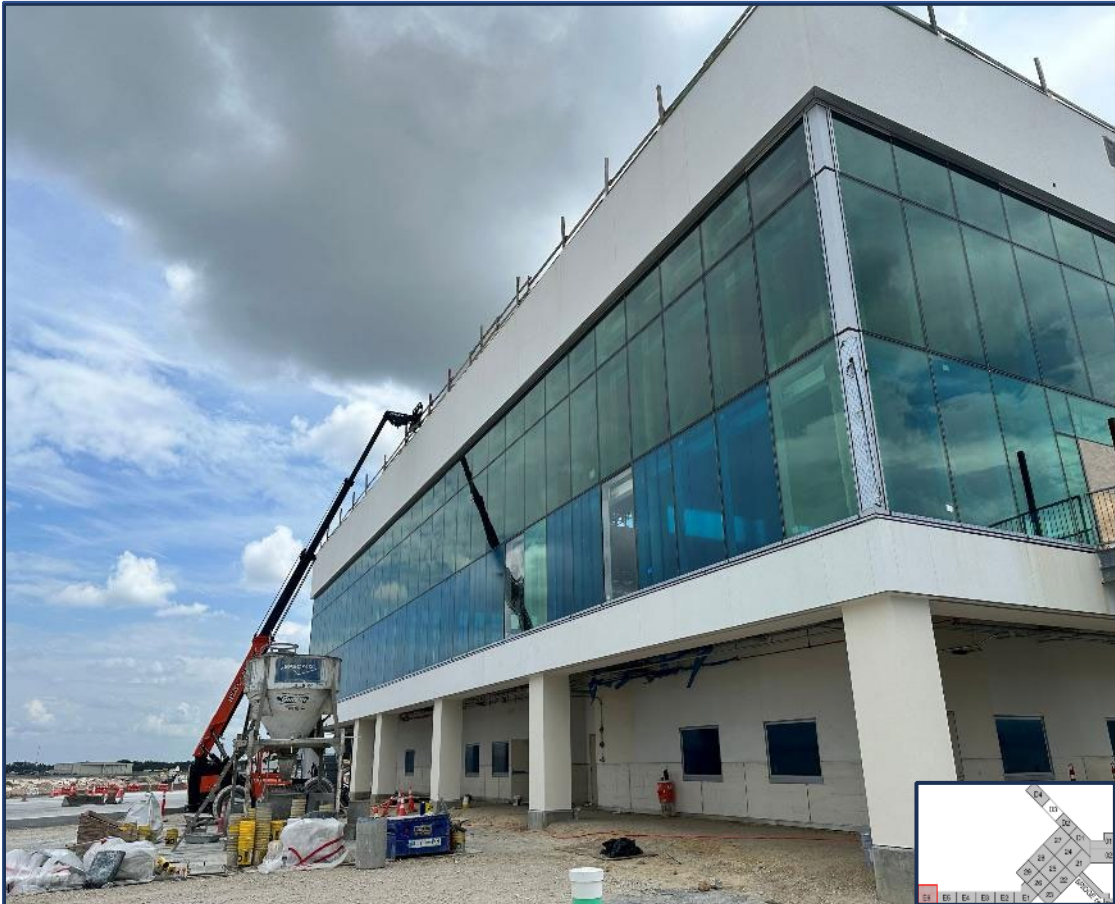
Curtainwall Installation in Zone E6 of Concourse E
