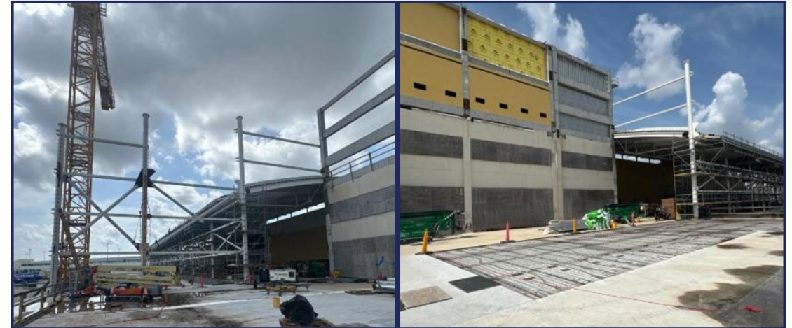
East and West High Arch Roof Trusses - Erection Started
