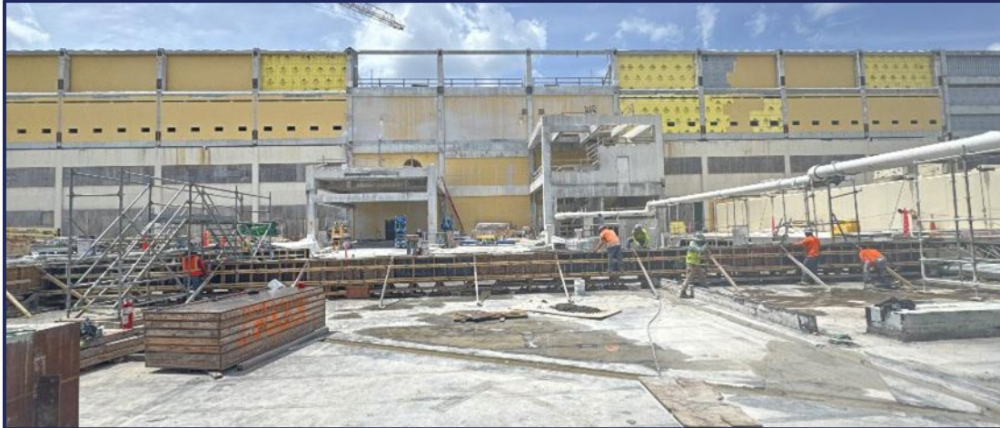
Concourse C Partial Demolition in Progress
