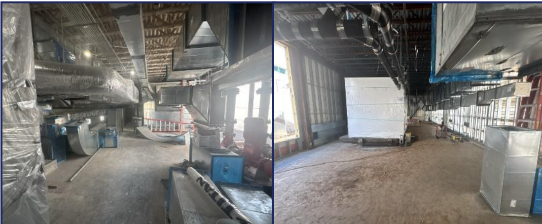
East and West Mechanical Penthouse Installations Continue
