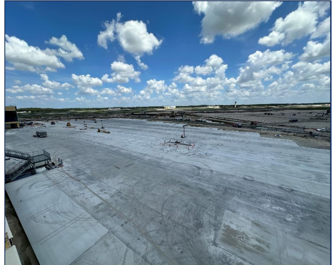
Continuation of concrete apron on the north side of Concourse E
