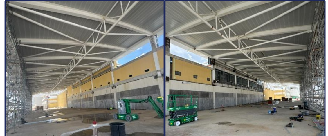
East and West Low Arch Roof Trusses and Epic Deck Installed
