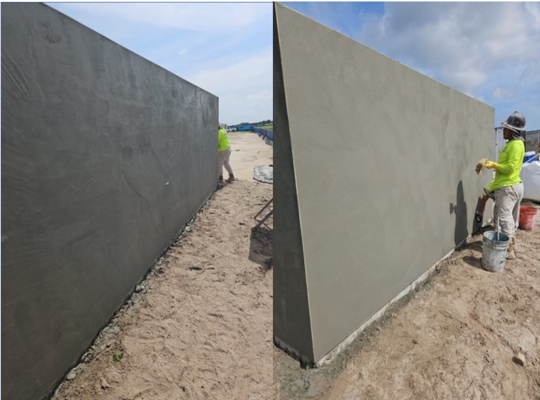
Stucco of the new dumpster enclosure was completed
