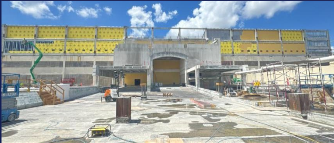
Concourse C Partial Demolition in Progress
