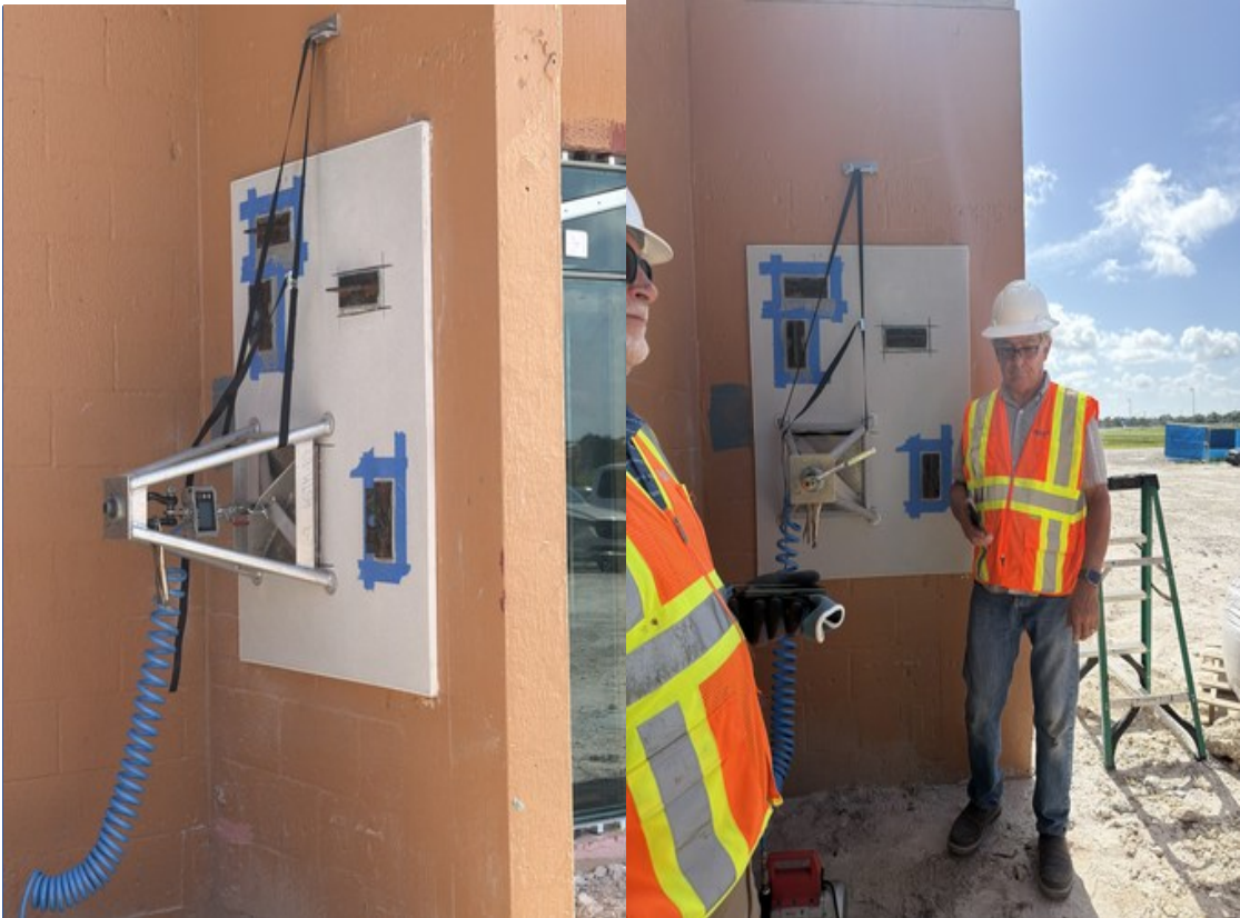
Stucco mockup was completed and passed the supplier's pull testing requirements
