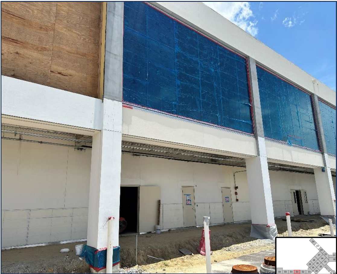
Continuation of stucco finishes and glazing on the south side of Zone E3
