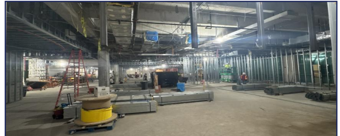
East Side Consolidated Checkpoint – Structural and MEP Underway
